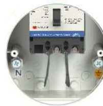
Internal zero and ground terminals Φ8 euro type connection handle
